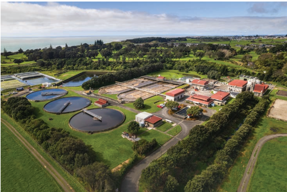
New Plymouth Wastewater Treatment Plant.
